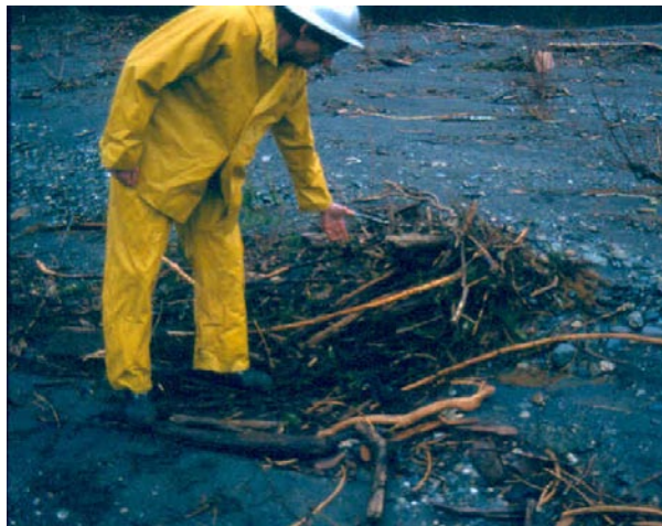
FIGURE 18.37 Live gravel bar staking traps small woody debris, creating a flow disruption and allowing sediment to collect (March 12, 1999). (Photo: D. Polster)
