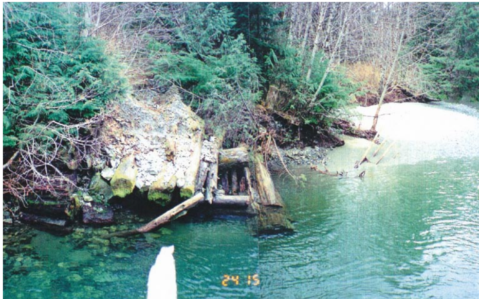
FIGURE 18.52 An old crib has distorted and settled, creating a scour pool in front of the logs; a gravel bar has developed on the downstream side of the collapsed crib. (Photo: G. Horel)
