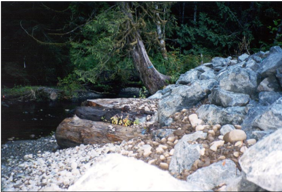
FIGURE 18.45 Habitat complexity was added to this channel by varying the alignment of the streamside face of the revetment and by anchoring large woody debris into the revetment. (Photo: G. Horel)
