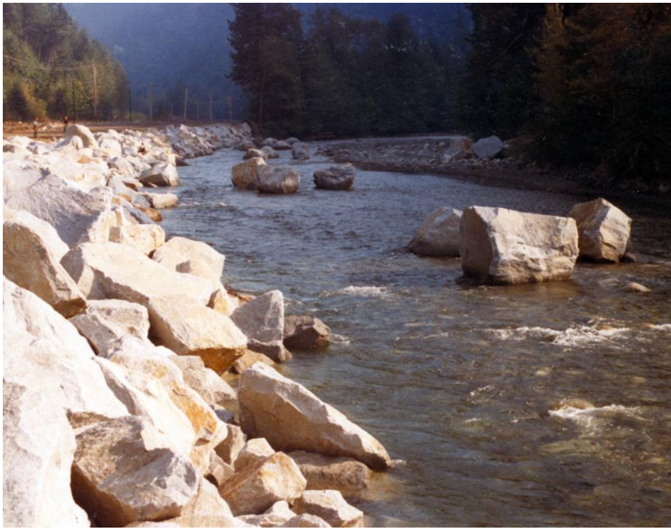
FIGURE 18.42 Coquihalla River, 1984: these boulder structures were constructed along the Coquihalla River using the largest rocks that could be moved with highway construction equipment. (Photo: M. Miles)
