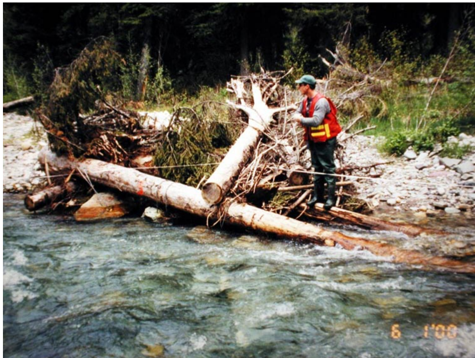
FIGURE 18.50 This large woody debris structure was constructed to narrow and deepen a degraded channel and provide fish habitat. (Photo: M. Miles)
