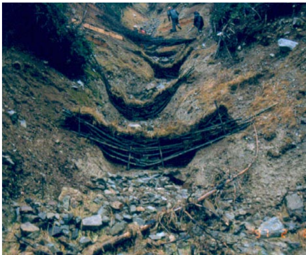
FIGURE 18.25 Live gully breaks can slow flows down gullies and promote recovery. Right photo shows treatment with water flows. (Photos: D. Polster)
