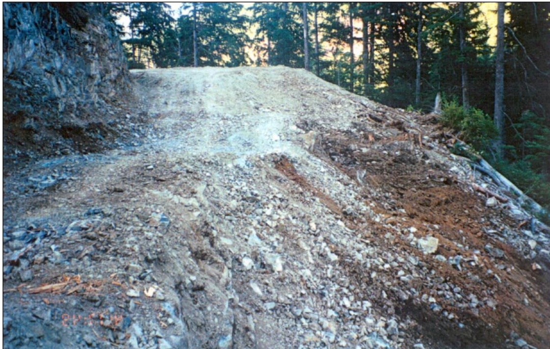
FIGURE 18.12 Fillslope instability has been substantially reduced by fill retrieval and endhaul; however, the remaining road surface is narrower. (Photo: D. Ostapowich)
