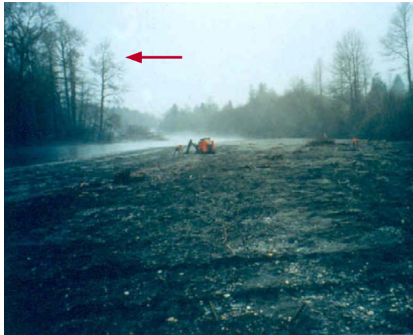
FIGURE 18.35 Live gravel bar staking on the San Juan River, March 12, 1998. The red arrow indicates a reference cottonwood. (Photo: G. Switzer)
