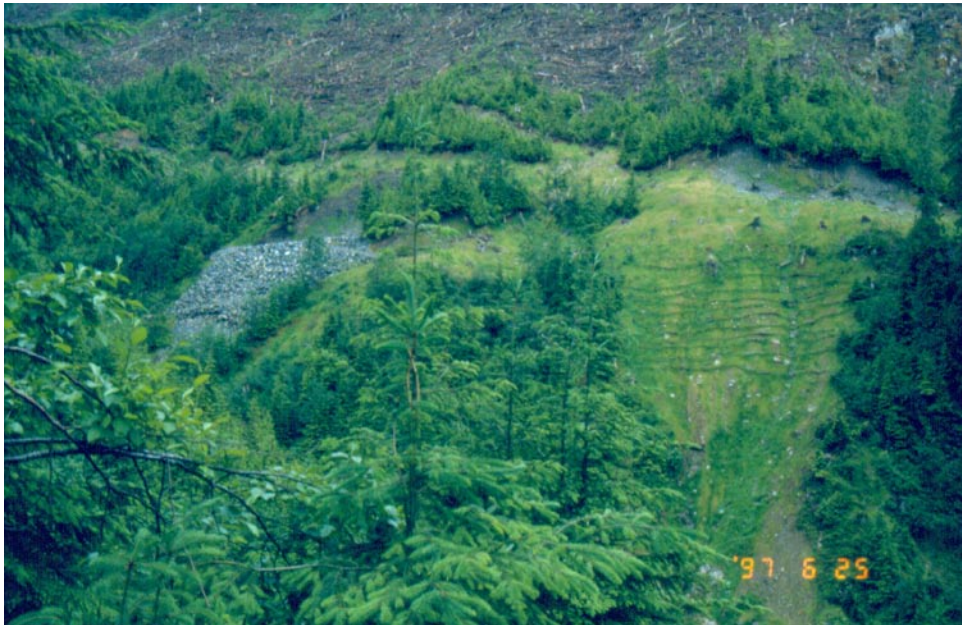
FIGURE 18.11 Soil bioengineering was used on this landslide to initiate the natural successional processes that will maintain a vegetation cover on this slope. The rock basin shown in Figure 18.10 can be seen on the left in this photo. (Photo: D. Polster)
