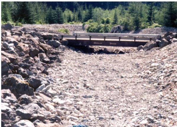
FIGURE 18.13 Low-level bridge on active mainline, designed to be overtopped during major floods or debris flow events. Tyler Creek, south central Vancouver Island. (Photos: G. Horel)
