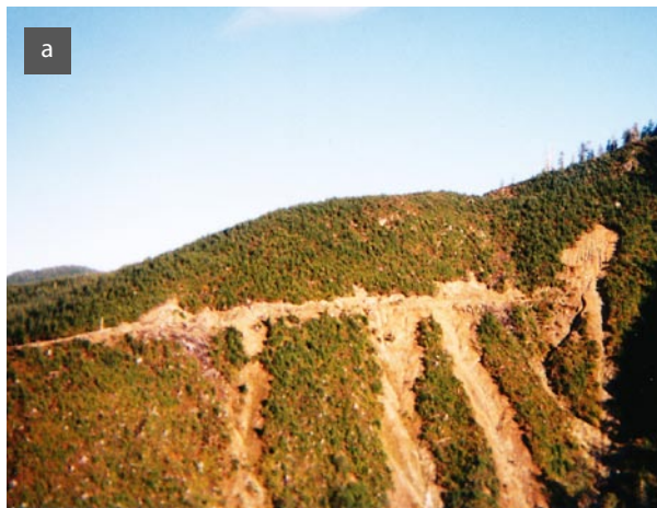
FIGURE 18.19 (a) Unstable fills and steep escarpments along a road section above Kennedy Lake on Vancouver Island. Road access to site was cut off by a large landslide (not visible). (b) Surface blast used to remove fill and trim landslide scarps. Photo shows site after blasting. (Archive photo from MacMillan Bloedel Limited, Kennedy Lake Division)
