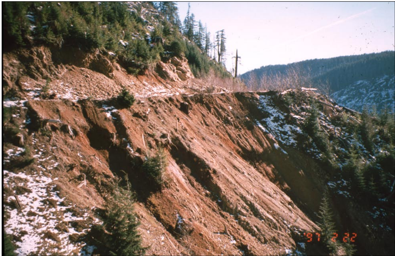
FIGURE 18.6 Example of road fill landslide, West Coast Vancouver Island. (Photo: T. Millard)
