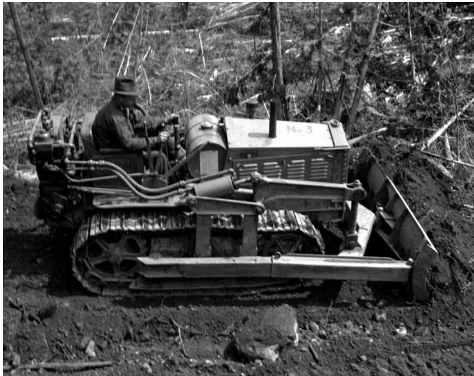
FIGURE 5.11 Bulldozers became popular in the 1940s, but their ability to sort materials on subgrade construction was not a strong feature. Bulldozers were one of the first road-building machines to add hydraulic components (the blade and winch). (Photo: Royal BC Museum Archives, NA-06355)
