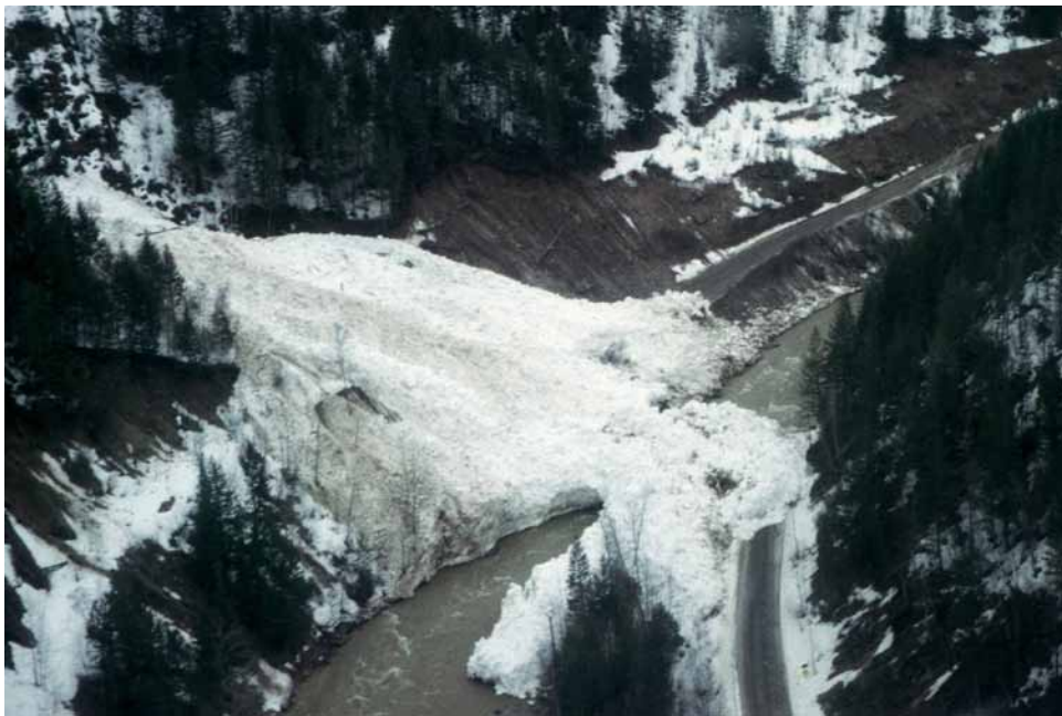
FIGURE 9.44 Bridge on Bull River in the Cranbrook Forest District destroyed in 1997 by a large avalanche in an established track. (Photo: D. Toews)
