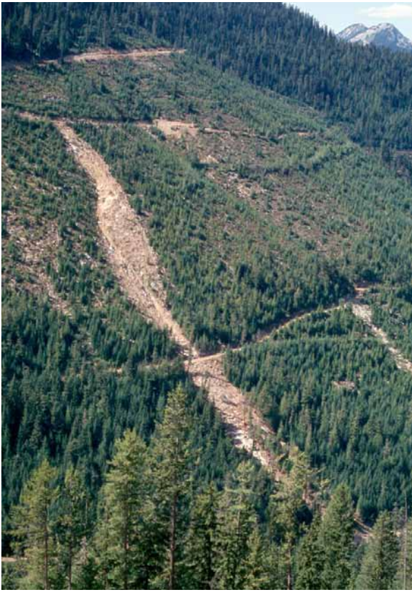
FIGURE 9.10 Debris avalanches (1993) caused by road-fill failures and drainage diversions on slopes logged in the 1970s at Airy Creek in the Arrow Forest District. (Photo: P. Jordan)
