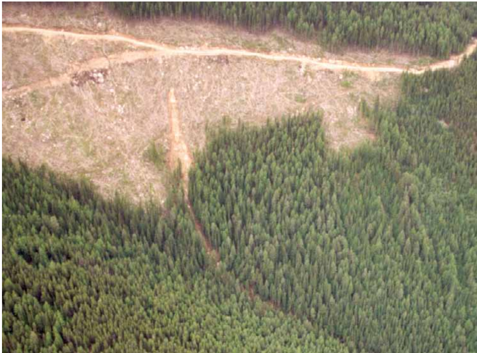
FIGURE 9.12 Debris slide that progressed to a large debris flow below a culvert in the Blueberry Creek area of the Arrow Forest District, 1993. The slide happened the spring following logging, occurring below a culvert that was misplaced by only a few metres from its optimum location. (Photo: P. Jordan)
