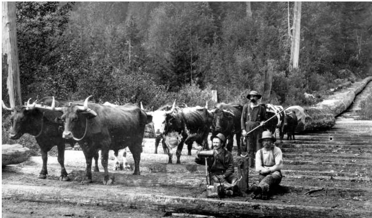
FIGURE 5.3 Skid road with log “skids” laid perpendicular to the direction of haul (circa 1890). (Photo: Royal BC Museum Archives, B-03827)
