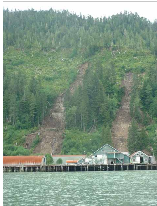
FIGURE 8.11 Shallow debris slides near Prince Rupert. (Photo: J.W. Schwab)
