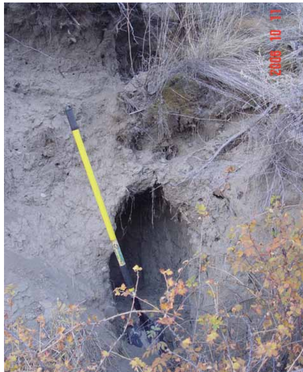
FIGURE 8.41 Pipe exposed on a bank of the Chilcotin River. (Photo: M. Geertsema)
