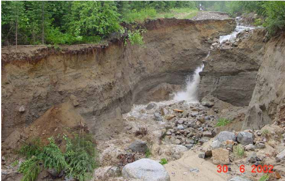
FIGURE 9.30 An extreme example of road erosion in the Lemon Creek drainage, Arrow Forest District, caused by diversion of a small creek down an old road during spring runoff (2002). (Photo: C. Pettitt, Valhalla Wilderness Society)
