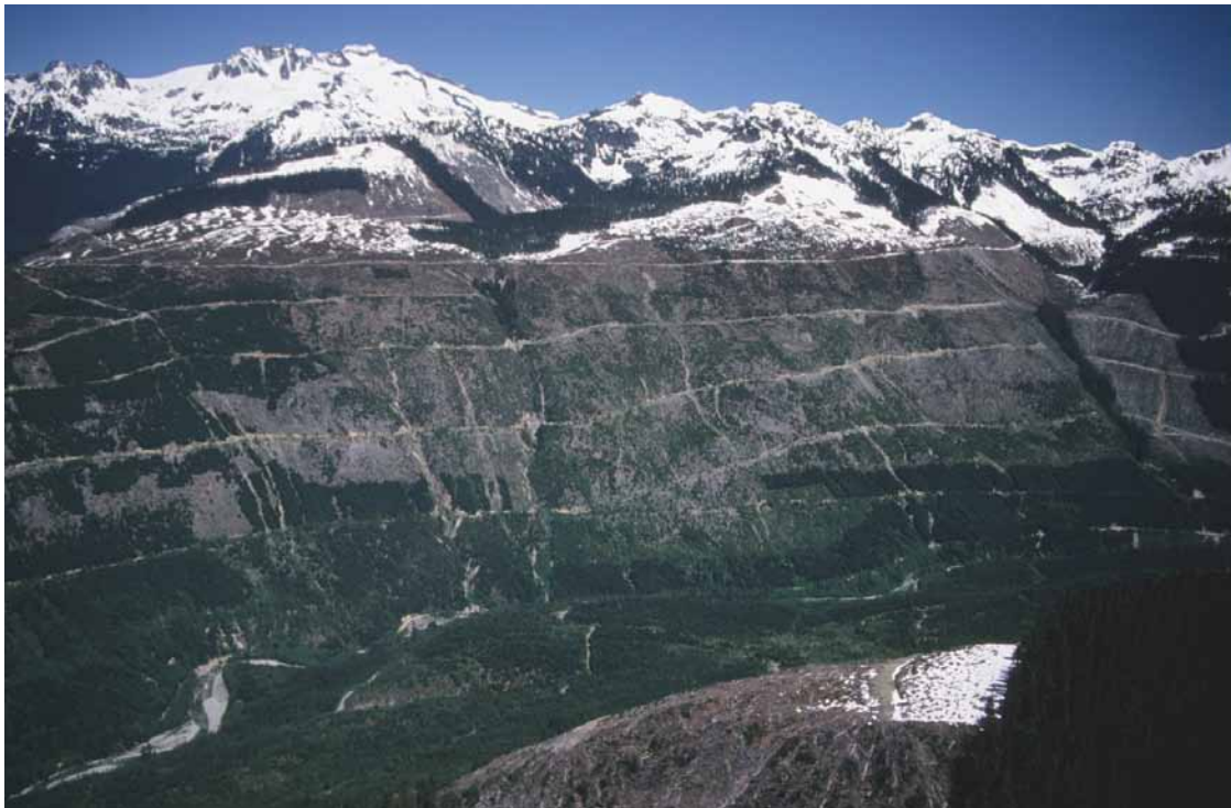
FIGURE 9.2 Numerous landslides caused by road-fill failure and harvesting effects in an area that was heavily logged in the 1970s. Many slides occurred 10 years or more after logging or construction. Mamquam River, Squamish Forest District. (Photo: P. Jordan)
