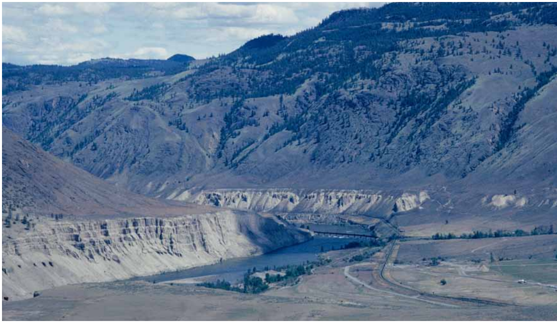
FIGURE 2.18 View upstream in Thompson Valley from Elephant Hill (Ashcroft). Colluvial cones overlie glaciolacustrine silts in the valley. The silts are prone to piping and mass failure when wet; significant landslides followed the inception of irrigated agriculture on the terraces. (Photo: J.M. Ryder)
