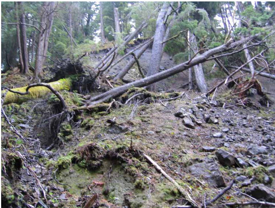
FIGURE 9.34 Unstable gully sidewall area in Rennell Sound, Haida Gwaii Forest District. (Photo: T. Millard)
