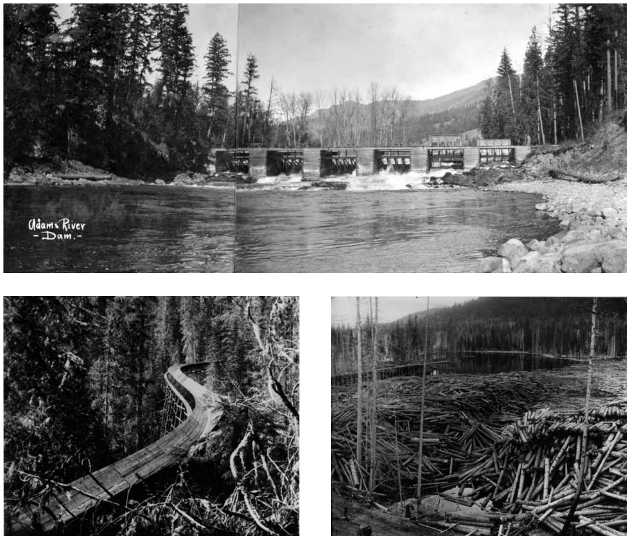
FIGURE 5.5 River transportation of logs on the Adams River: the Adams River splash dam (top), Brennan Creek flume (bottom left), and Adams Lake sorting pond filled with logs to be driven down the Adams River (bottom right). (Photos: Royal BC Museum Archives, I-62756, F-09177, F-09179)
