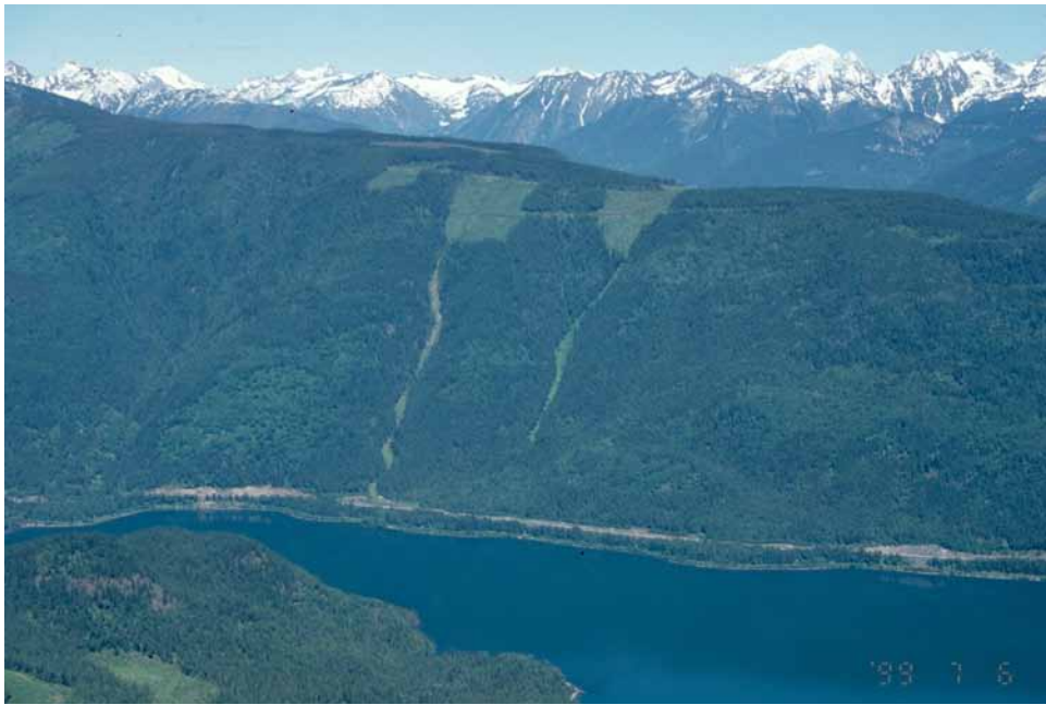
FIGURE 9.43 Avalanches in these two cutblocks in 1988 created avalanche tracks that threaten the highway below on Slocan Lake in the Arrow Forest District. (Photo: P. Jordan)
