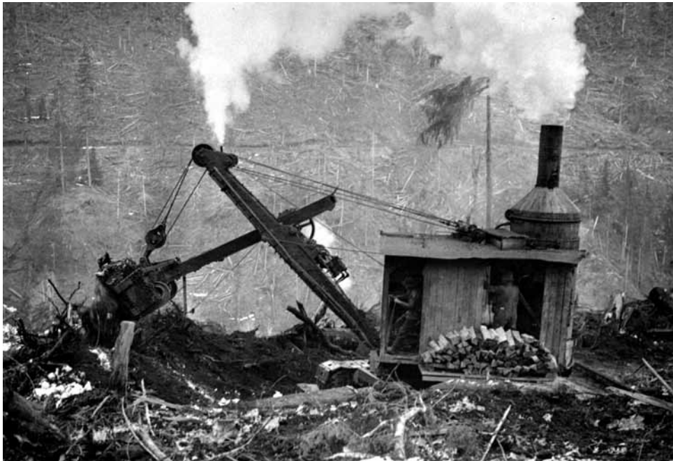
FIGURE 5.9 Wood-burning steam shovel near Cowichan Lake in 1935. (Photo: Royal BC Museum Archives, H-05397)
