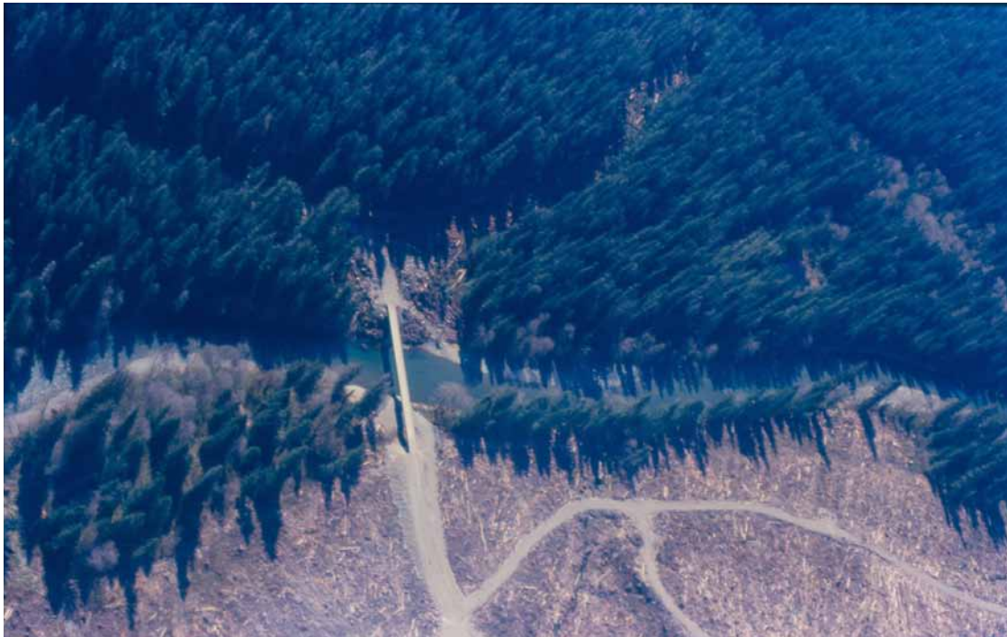
FIGURE 5.16 The use of steel girders has allowed for longer spans without obstructions to water flow (Klanawa River). (Photo: D. Bendickson)
