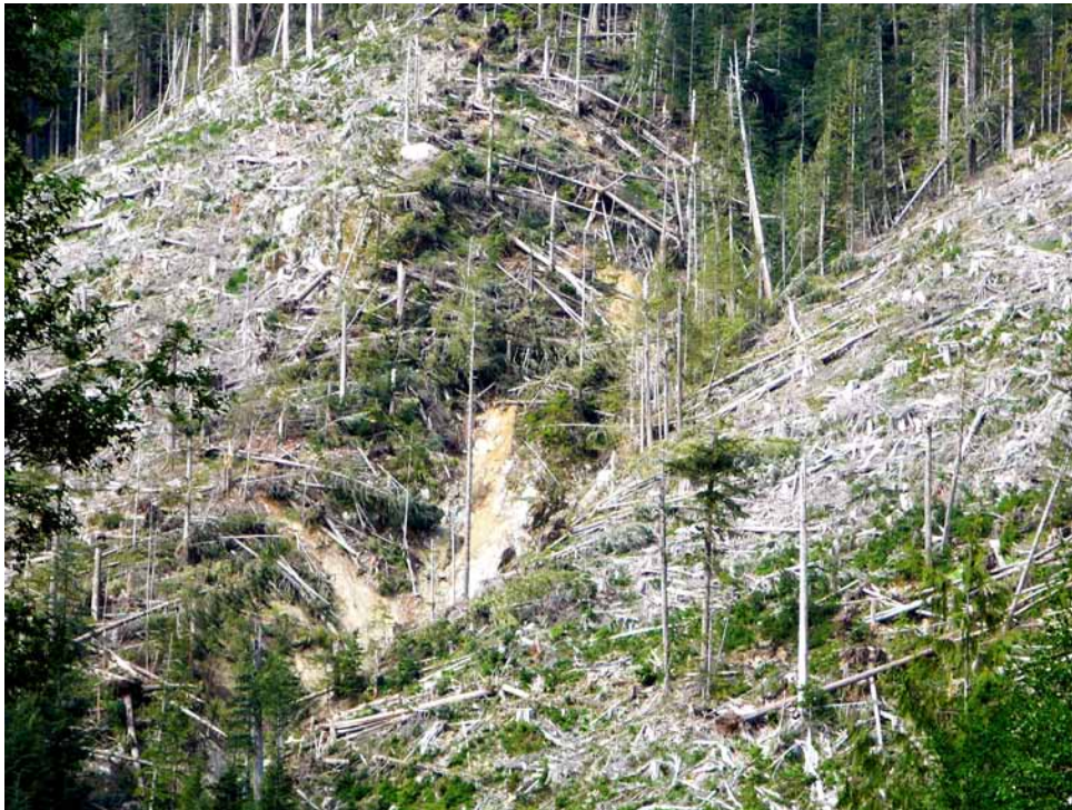
FIGURE 9.36 Debris slides in a gully near the Klanawa River in the South Island Forest District. The gully was left unlogged but was heavily damaged by windthrow. (Photo: T. Millard)
