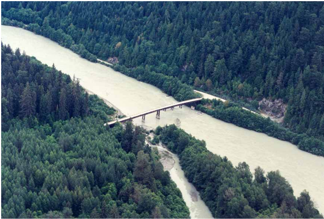
FIGURE 5.15 The bridge over the lower Klinaklini River illustrates a “glulam” bridge with simple spans and a longer inverted truss span. (Photo: D. Bendickson)
