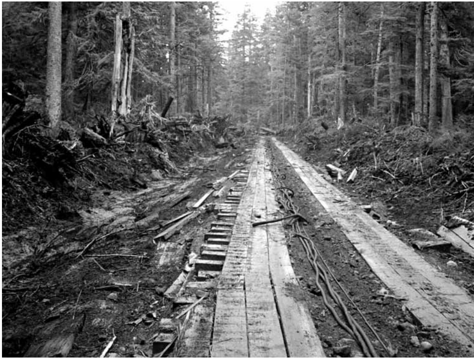
FIGURE 5.8 Excavating deep organic soils and hauling ballast for roads could be prohibitively expensive compared to building plank roads. Some of these roads were built over railroad grades by replacing the steel rails with planks. (Photo: Royal BC Museum Archives, NA-08441)
