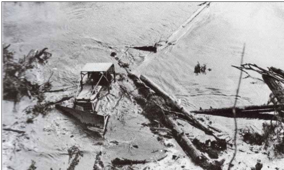
FIGURE 5.12 Moving water (in any volume) is an inconvenience to road construction because it requires some form of a special structure to span it. Before stream morphology was commonly understood, moving water was generally viewed as “self cleaning.” (Photo: Gould 1975, reproduced with permission of Hancock House Publishers)
