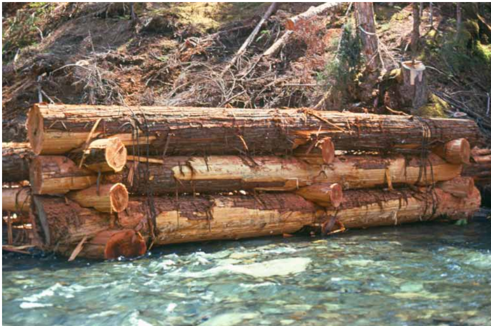
FIGURE 5.14 Because of span limitations for log-stringer bridges, the footing structures often intruded into the wetted perimeter of the creek. Scouring associated with such construction was an ongoing problem. Moakwa Creek (Upper White River tributary) circa 1972. (Photo: D. Bendickson)
