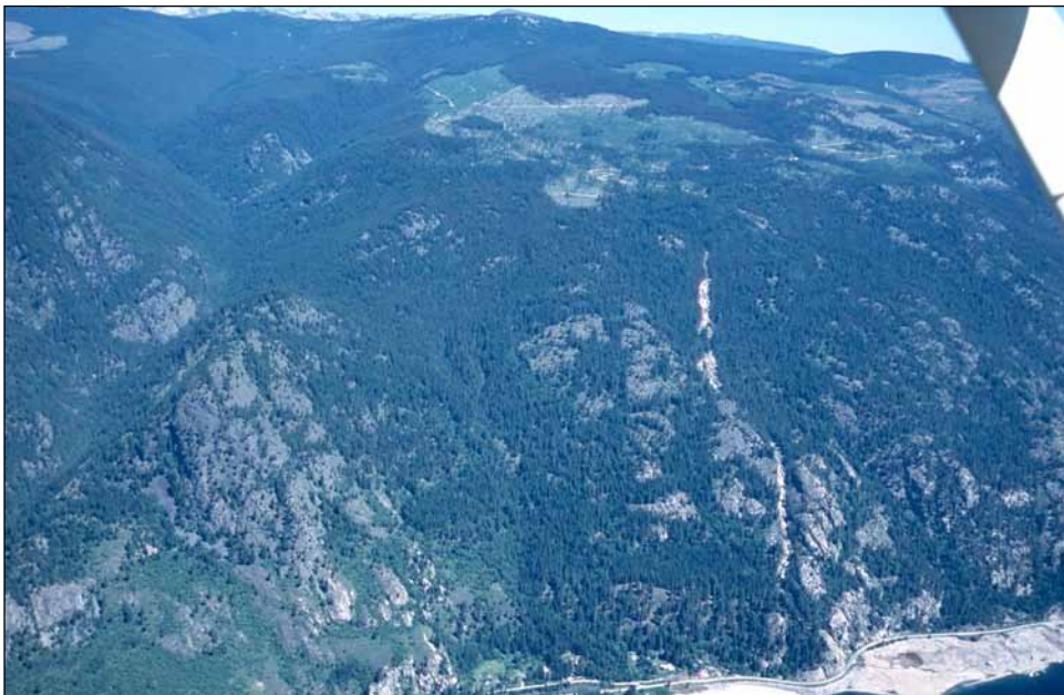
FIGURE 9.20 "Gentle-over-steep" debris flow caused by road drainage diversion on Lower Arrow Lake in the Arrow Forest District, 1999. On a newly constructed road, two culverts were not installed on a small ephemeral stream, and water was discharged off a switchback. This caused the debris flow, which began as a small debris slide below the switchback. (Photo: P. Jordan)
